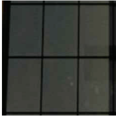
STANDARD BRONZE ANODIZED ALUMINUM STOREFRONT SYSTEM WITH 1" INSULATED CLEAR GLAZING
